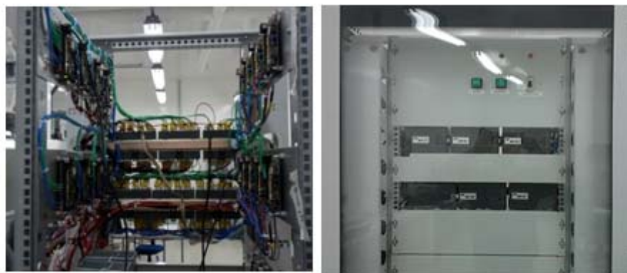
Fig. 5 Siemens Programmable Logic Controller (PLC) and stepper motor drivers to control machines and processes for Iodine-125 seeds quality controls.
