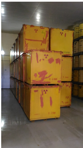
Figure 3 - Boxes with waste from the Goiânia accident today. The stains are scratches on the painting and corrosion points that were fixed.
