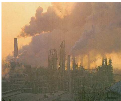
Flue gas Purification
