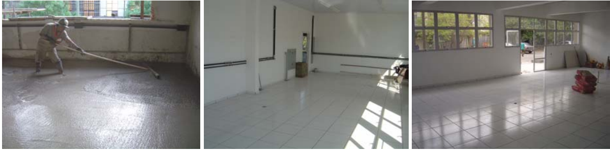
Figure 4: The new laboratories of CQMA after rebuilding.
