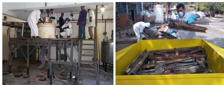
Figure 2: Dismantling operations of the ADU Dissolution and Uranyl Nitrate Purification Pilot Plants.
