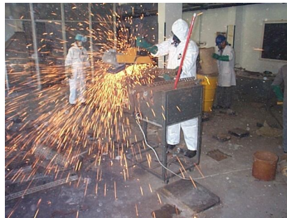
Figure 9. Cutting operation using an abrasive disc in a stationary machine.
