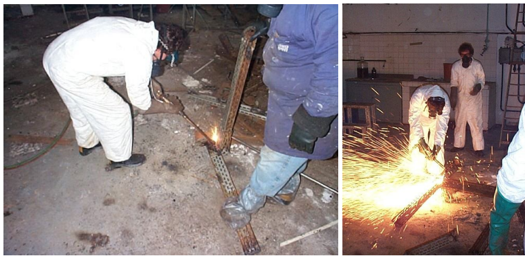
Figure 2. Segmentation of carbon steel structures using an oxygen-acetylene torch [4, 5].
