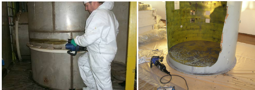
Figure 4. Tanks cutting using a nibbler [6-8].
