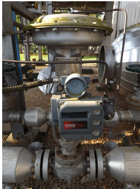
Figure 1. Control valve and the inteligente positioner.
