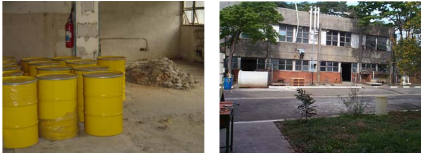
Figure 6: Contaminated layer removal and external view of the facility.
