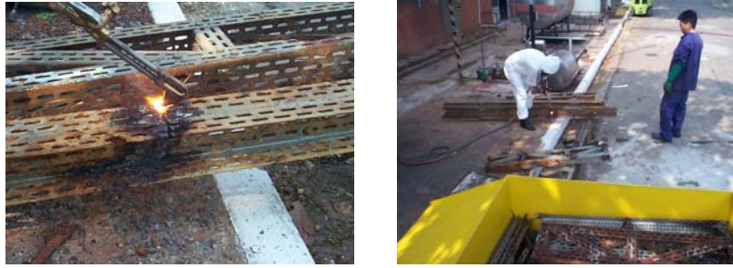
Figure 2: Structure cutting with oxyacetylene torch and storage in steel box.
