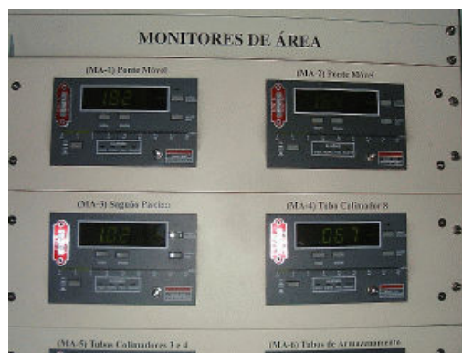
Figure 1 Area Monitors modules (MA1 to MA4) located in the reactor control room
