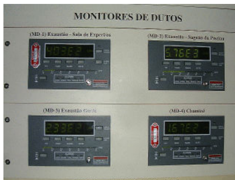
Figure 2 Duct monitors modules (MD1 to MD4) located in the reactor control room
