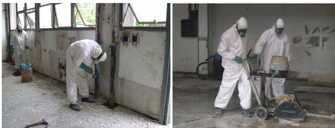
Figure 3: Decontamination tasks on the wall and humid method for the floor.
