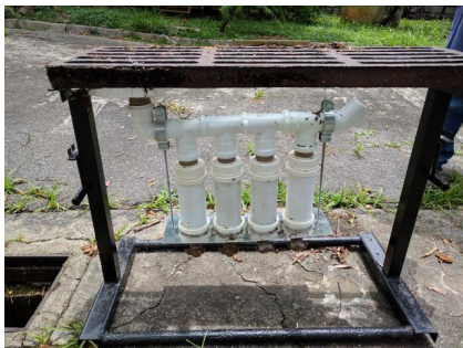
Fig. 1. Integrated Collector built with PVC tubes (adapted from [1, 9]).
