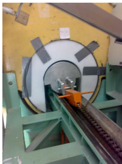
Figure 3 – Polyethylene shielding piece a the BNCT facility beam hole
