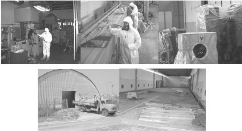
Figure. 2: In this picture there are, respectively, the monitoring, the disassembly, the packing and labeling of materials in the building 24, and finally the transportation and the installation of this planned operation.
