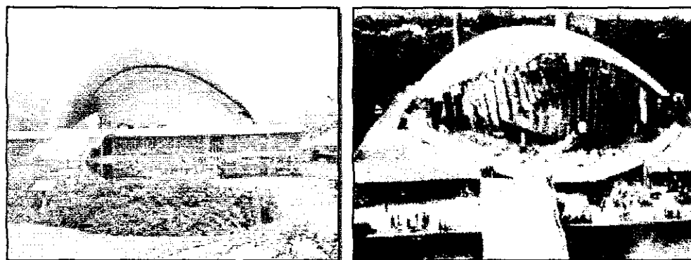
Figura 1.4 – O Colapso do Berlin Congress Hall 7 .
