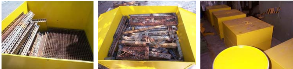
Figure 12: Contaminated structural parts of carbon steel stored in steel boxes (left and center) and storage of the steel boxes with radioactive waste (right).
