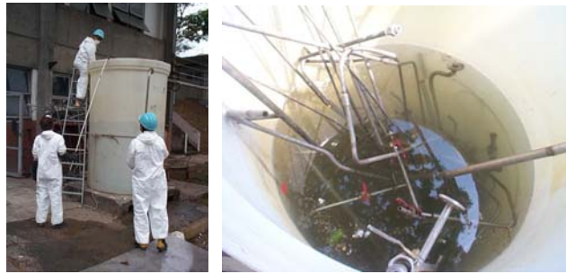
Figure 6: Polypropylene tank adapted for decontamination of large steel pieces.
