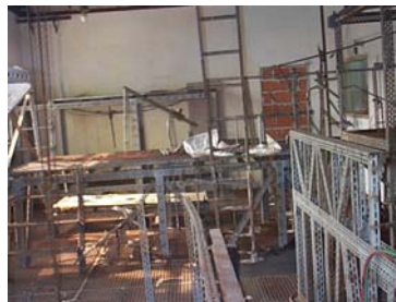
Figure 2: The same structure shown above after tanks and piping removal.
