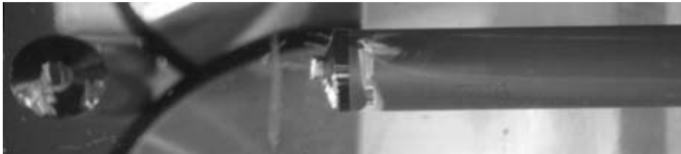
FIG. 9. Photographs of fuel leakage in welding joint in the reactor
