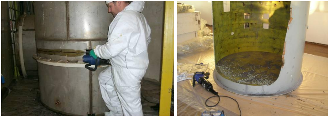
Fig. 4 Tanks cutting using a nibbler.
