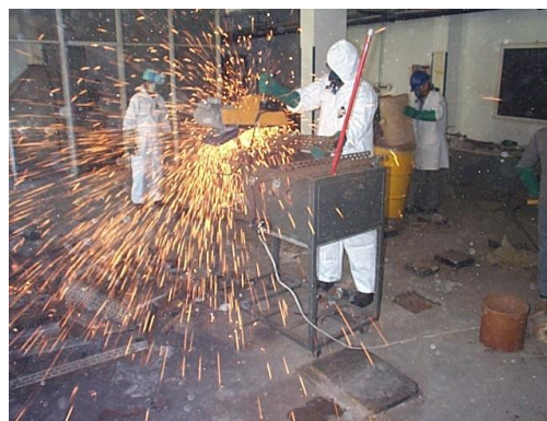
Fig. 9 Cutting operation using an abrasive disc in a stationary machine.
