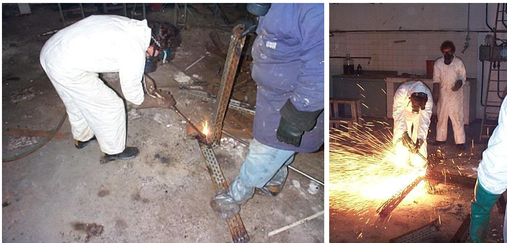
Fig. 2 Segmentation of carbon steel structures using an oxygen-acetylene torch.
