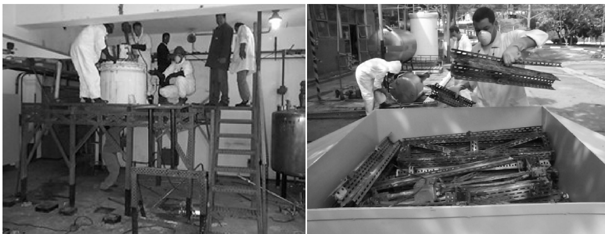
Fig. 2 Some pictures of dismantling operations of the ADU dissolution and uranyl nitrate purification pilot plants.
