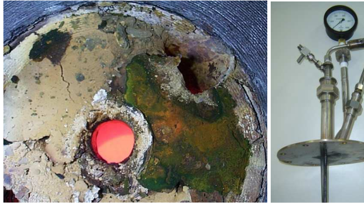
Figure 5: Clogging of salt solidified in the upper region of the reactor (left), molten salt can be observed through the central hole left by the injection lance (right).
